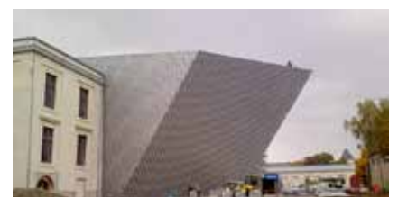
Profile sheet grids by Graepel are being used in the new design of the German Army's Museum of Military History in Dresden.
